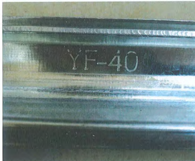
'YF-40' FLANGE CROSS JOINT
